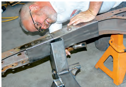
8) The crossmember was installed and it was a tight fit. A few hammer whacks were necessary to get the centerlines to match up.
