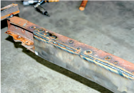
7) Here's what the framerail looked like after it was boxed. This strengthens the frame at the point where the crossmember will be installed. Without this, the frame could tear from stress over time.
