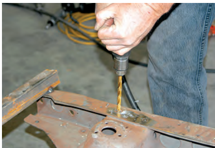
2) Using a 3/8-inch drill, the rivets were drilled to remove the shanks.
