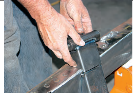
11) The upper A-arm mount or tower had to be installed next. It was placed on the frame and extends upward from the lower crossmember.
