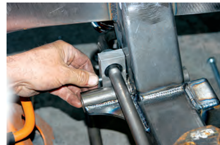
13) The Swaybar block was bolted to the crossmember on the bottom, and when it was in place, the upper bolt hole was drilled and tapped. Doing it this way ensures that the bolt holes will line up.
