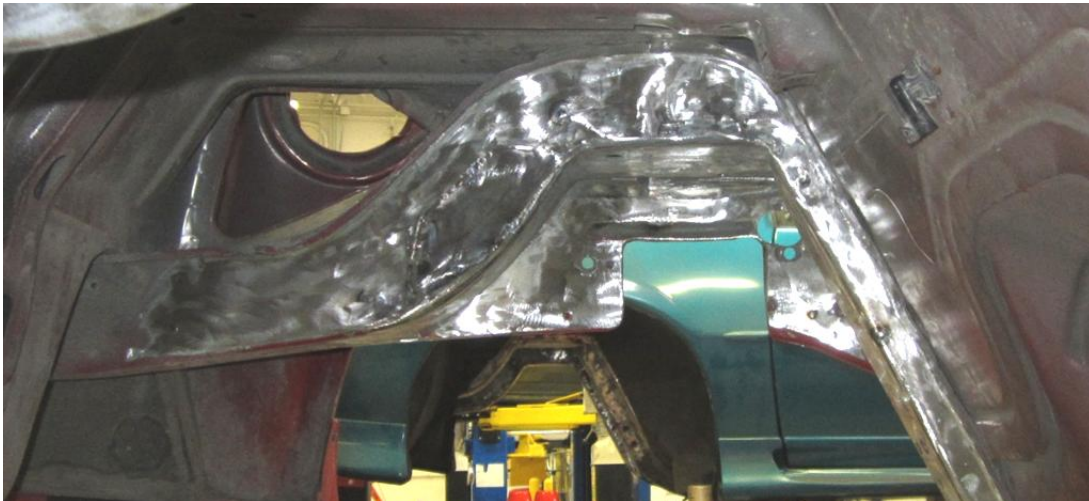
Inside View, Drivers Side, Upper Control Arm Cut-Out, Figure 57
