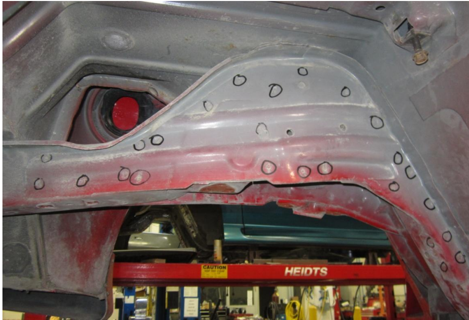
Drivers Side Inner Frame Rails, Mark Spot Welds, Figure 3
